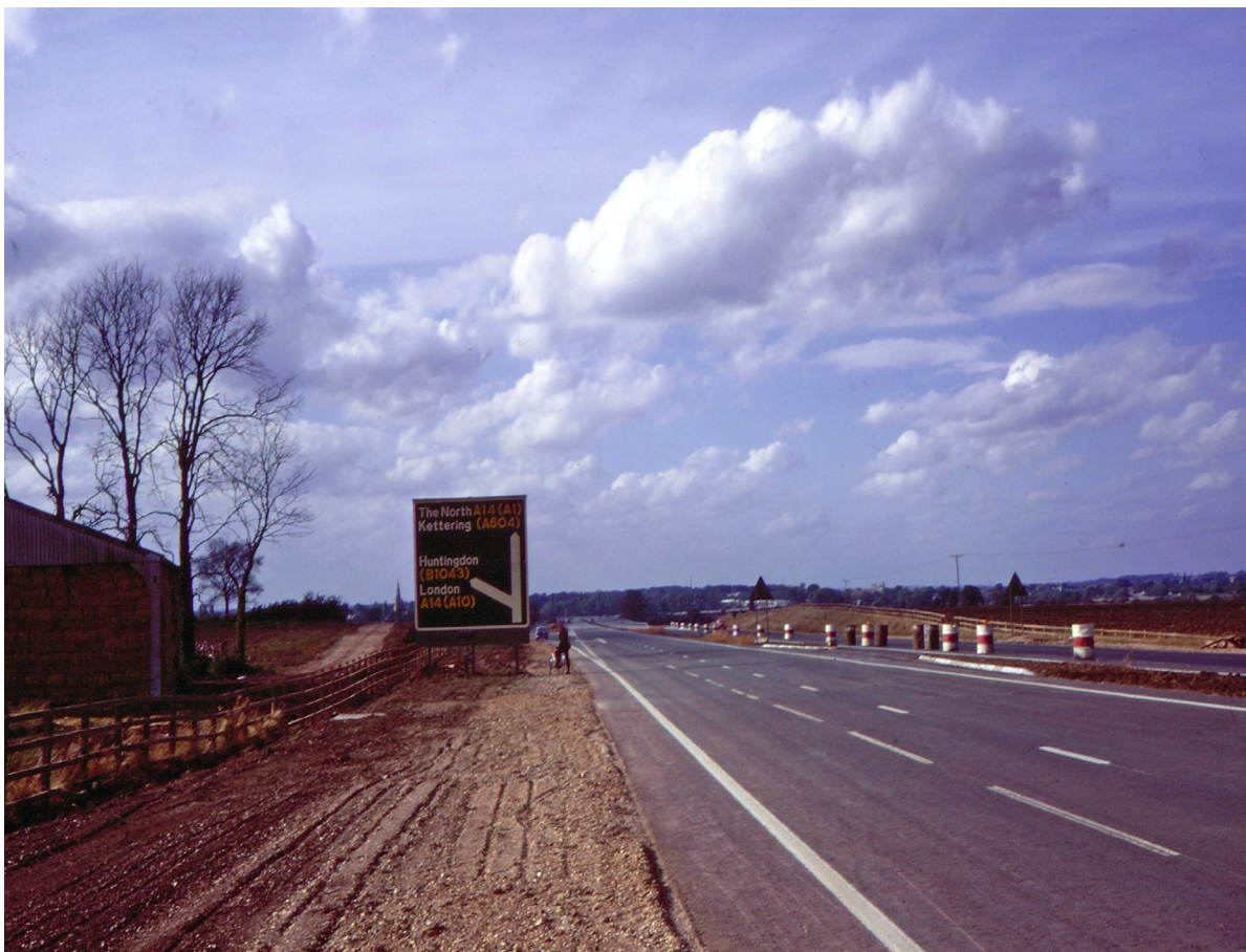
Figure 142: Here is the newly dualled road at the Godmanchester junction just before the official opening. An empty road – but not for long
