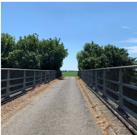
Figure 143: The 1981 Mere Way flyover of the old A14 giving access for the bridleway and Topfield Farm
