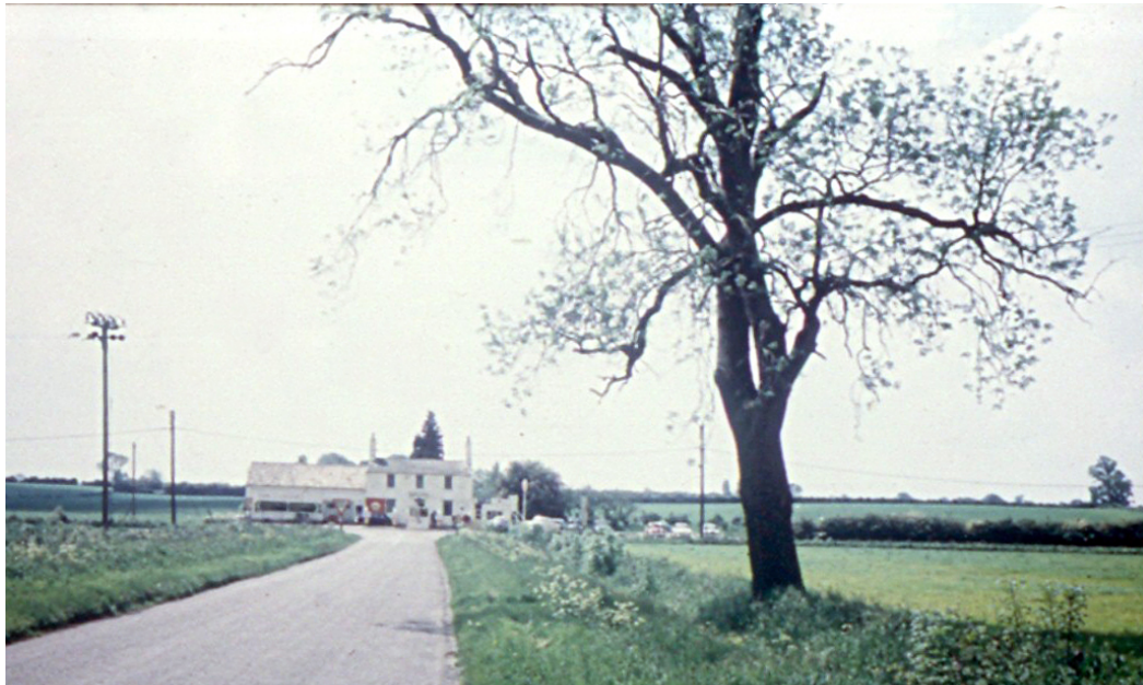
Figure 129: Looking south along Rideaway to the Lion Garage
