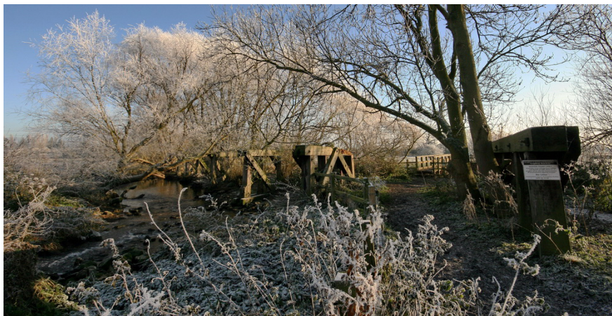
Figure 72: Wooden skeletons of the railway bridges at Houghton
