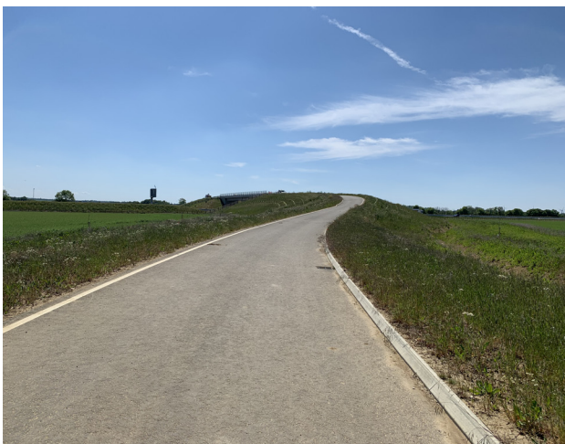
Figure 145: The second Mere Way bridleway and farm flyover. This crosses the new A14 close to Hilton
