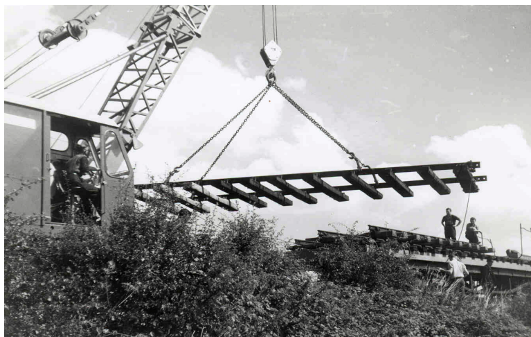
Figure 71: Lifting the tracks
