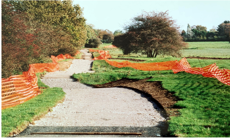
Figure 117: The cycleway under construction
